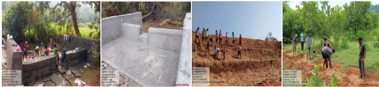
Fig: Check dams, Farm Pond & Field bund activities at different villages through MGNREGA
