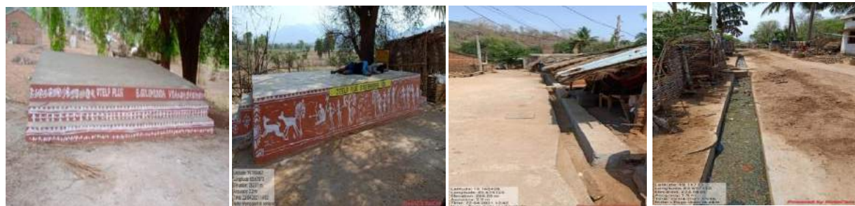
Fig: Construction of Drying Yards and Drains under EPA activities
