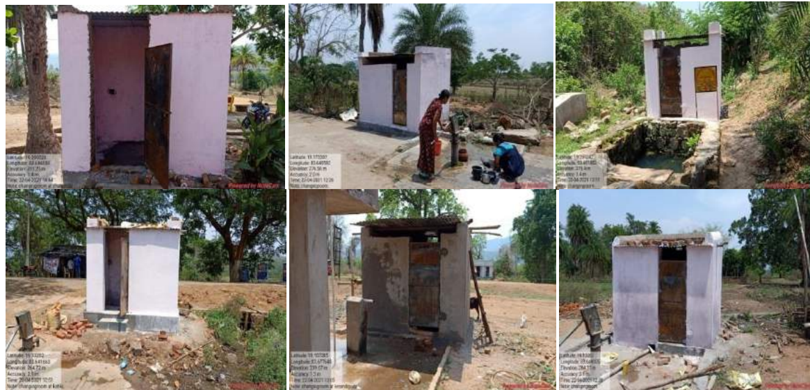
Fig: Construction of Changing rooms at different villages under EPA activities
