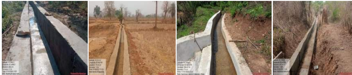
Fig: Machinery Canals at different villages through MGNREGA
