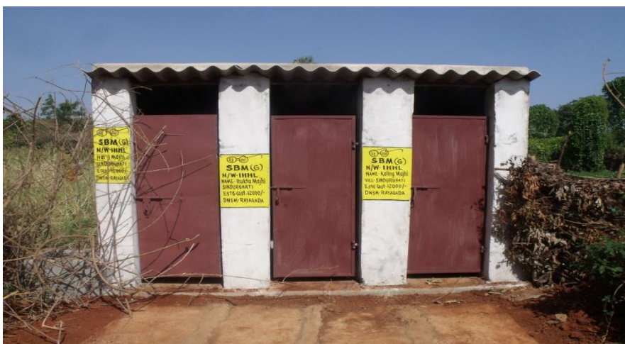
Fig:- Construction of IHHL at OTELP village
